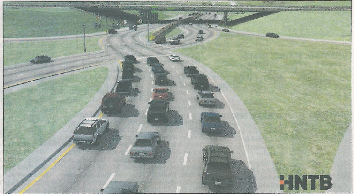
An illustration of a planned double crossover diamond interchange from Ky. 536, with Interstate 71/75 crossing overhead. Motorists would briefly switch to the opposite side of the road. KY. TRANSPORTATION CABINET
