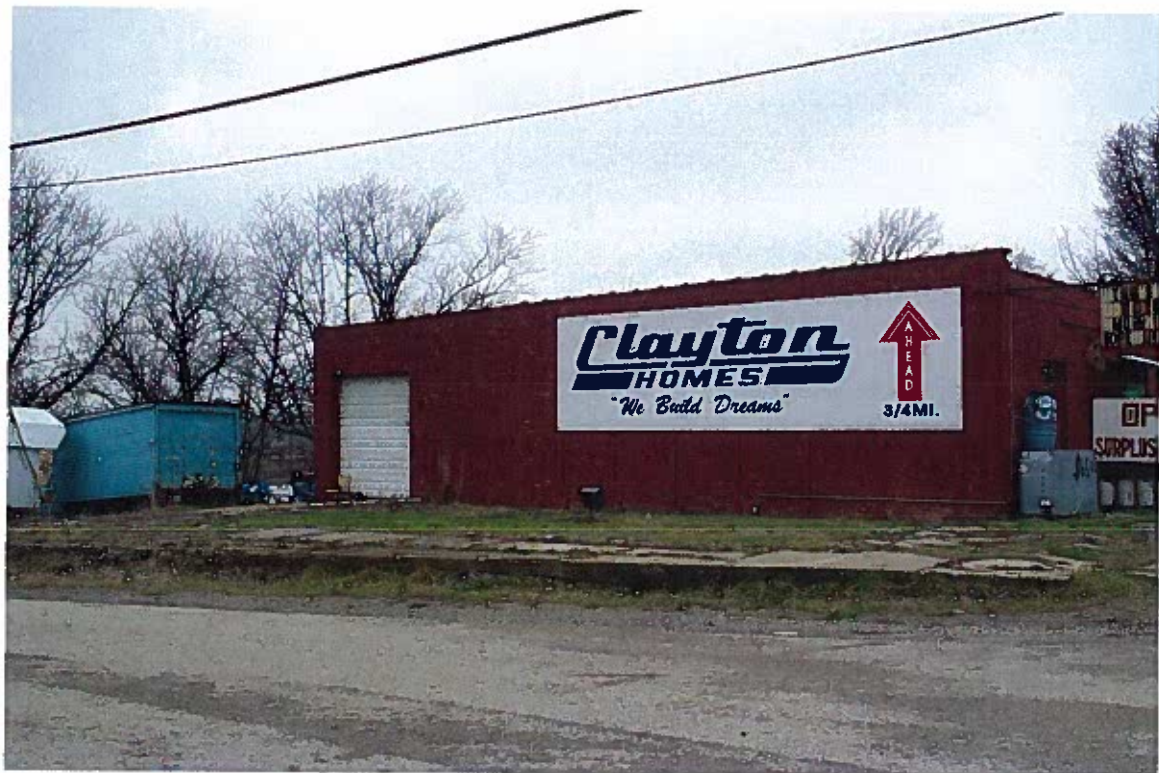
Figure 12. Site 9, Side elevation of Richwood store
